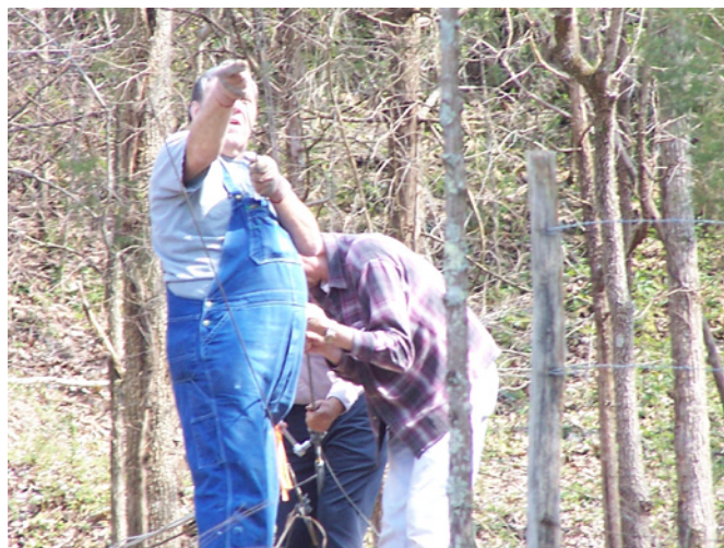
The ground crew of Wes, WJ4DX; Butch, K4MGB and myself had to keep a tight hand on the guys. They had to be loosened to allow the antenna to be raised over each guy point.
